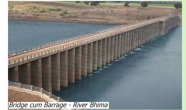
Bridge cum Barrage - River Bhima
