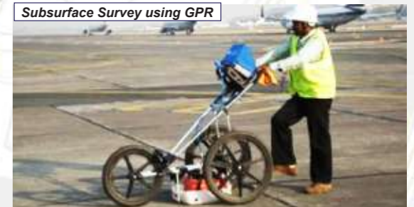
Subsurface Survey using GPR
