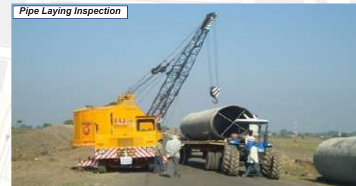
Pipe Laying Inspection
